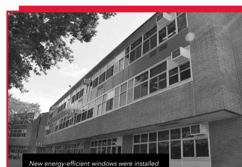
New energy-efficient windows were installed at Edmund W. Miles Middle School.
